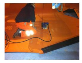
FLAGON PM/SL waterproofing membrane includes a thin coloured layer or "signal layer" on the visible side of the membrane which allows any damage to be immediately identified and repaired.
