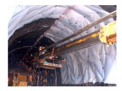
The sheets are welded together by applying hot air or using hot wedge, with manual or automatic welder. The welding can be made either with a track that with double track. The double track allow to perform a pneumatic test with air.
