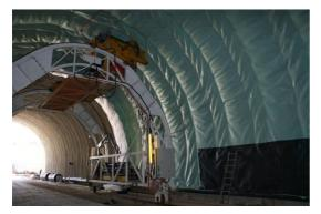
The waterproofing membrane FLAGON BSL includes a thin colored layer on the visible face of the membrane that allows a quick visual check of any damage occurred to the membrane during the application. This layer is called the "signal-to-layer".
